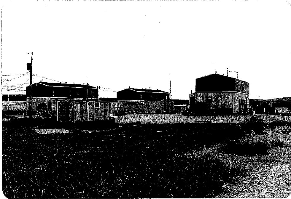
Photo 3. Planned location of sixplex in Zone B. View towards the southeast.
